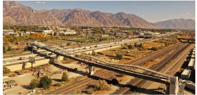
The new pedestrian bridge at the Utah Valley University is longer than three football fields. Photo courtesy of Uponor
