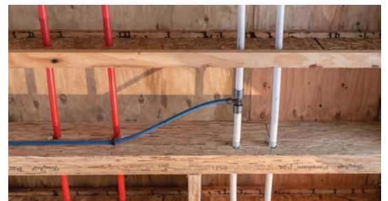
PEX plumbing installation in a multifamily project.
