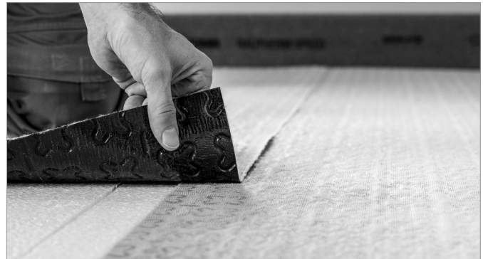
Fig 4.2 Overlap of 4 in (10 cm) on cross (perpendicular) edges
