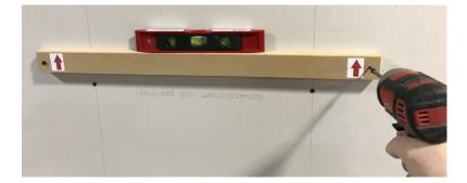
5. Mark the MDF strip with the centerline of the wall stud.
