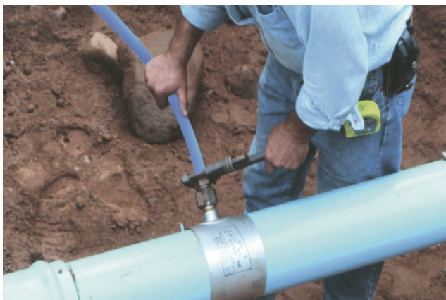
Fig. 10: Angle MUNICIPEX pipe 10 to 20° above horizontal at connection to main
