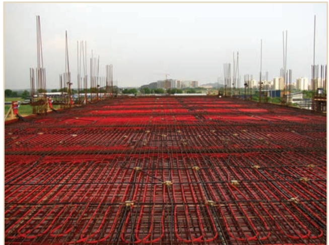
FIGURE 6: Radiant slab system before concrete pour.
