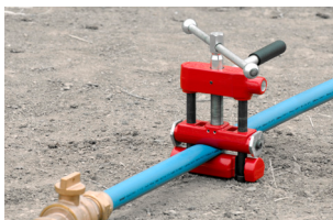
Fig. 12: Pipe in squeeze-off tool
