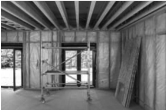
Fig. 2: Underside of joist space construction
