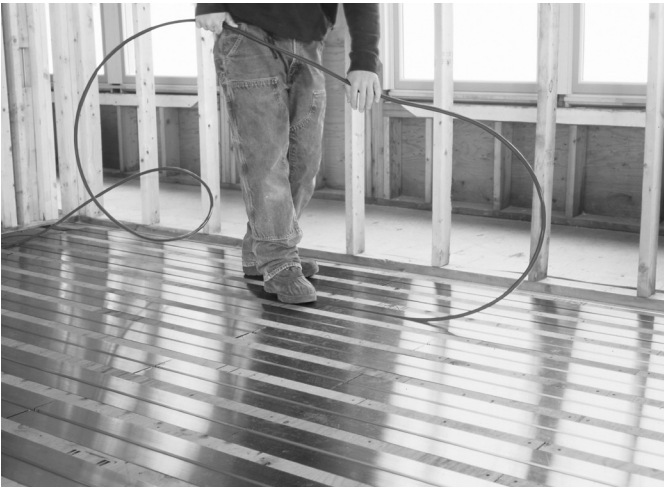
Fig. 1: Installing RAUPANEL to wood subfloor over joists
