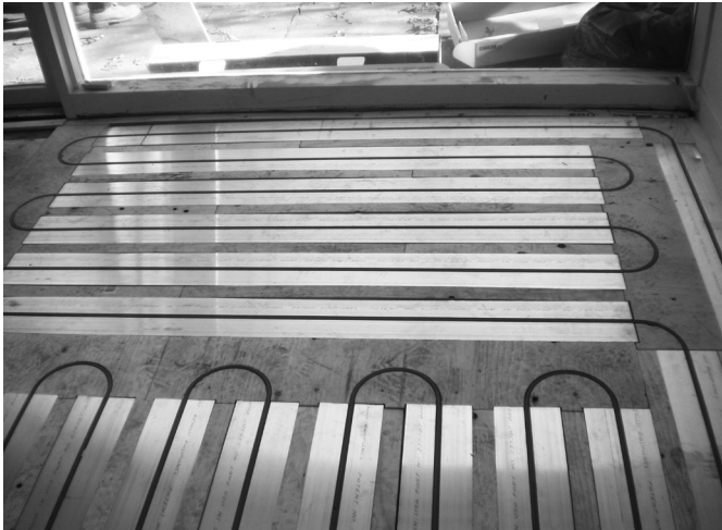
Fig. 6: Installing RAUPANEL with warmest water to the perimeter (an exterior door) then to the occupied (interior) areas of a room
