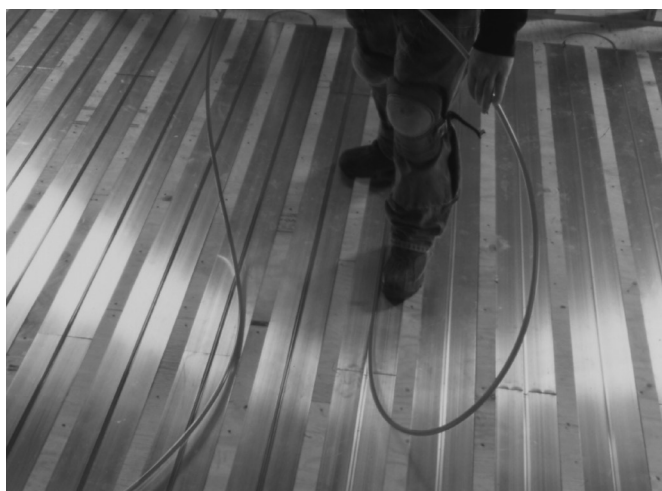
Fig. 15: Install pipe by stepping into groove with sole of work boot
