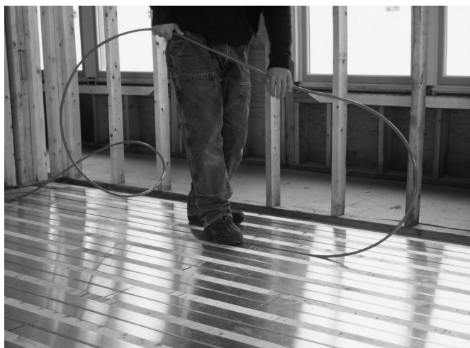
Fig. 24: Snapping pipe into groove
