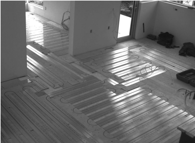
Fig. 5: Installing RAUPANEL with complex piping layouts
