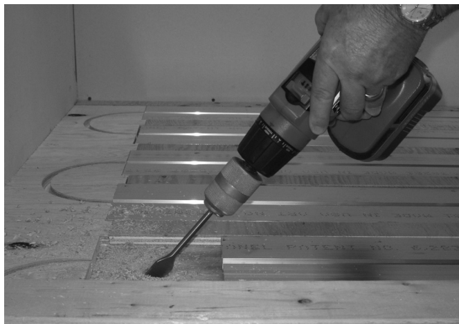
Fig. 23: Drilling subfloor penetrations for supply and return tails
