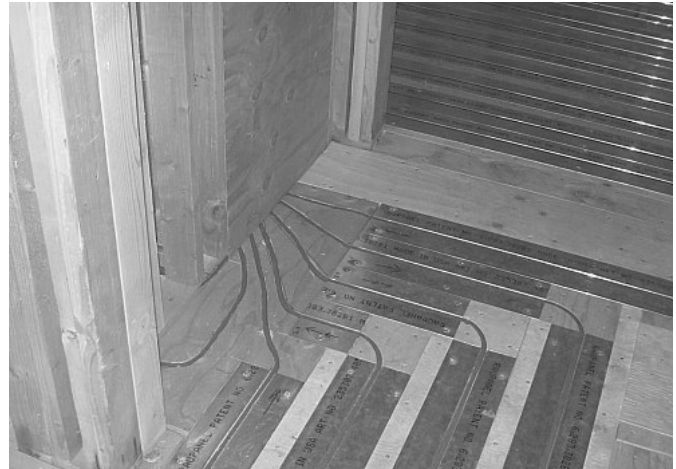
Fig. 17: Grooves custom-routed in plywood for supply and return tails
