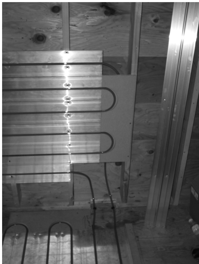
Fig. 20: Typical installation with tails routing into floor circuit
