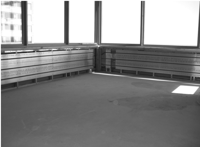
Fig. 2: Installing RAUPANEL to steel wall studs
