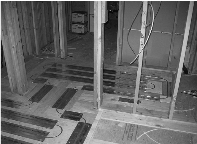
Fig. 4: Installing RAUPANEL through a doorway
