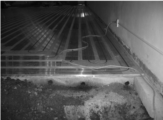
Fig. 3: Installing RAUPANEL directly above an existing slab
