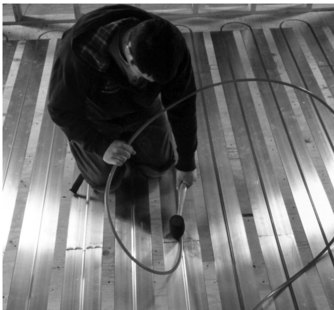
Fig. 21: Installing pipe by setting into groove with rubber mallet
