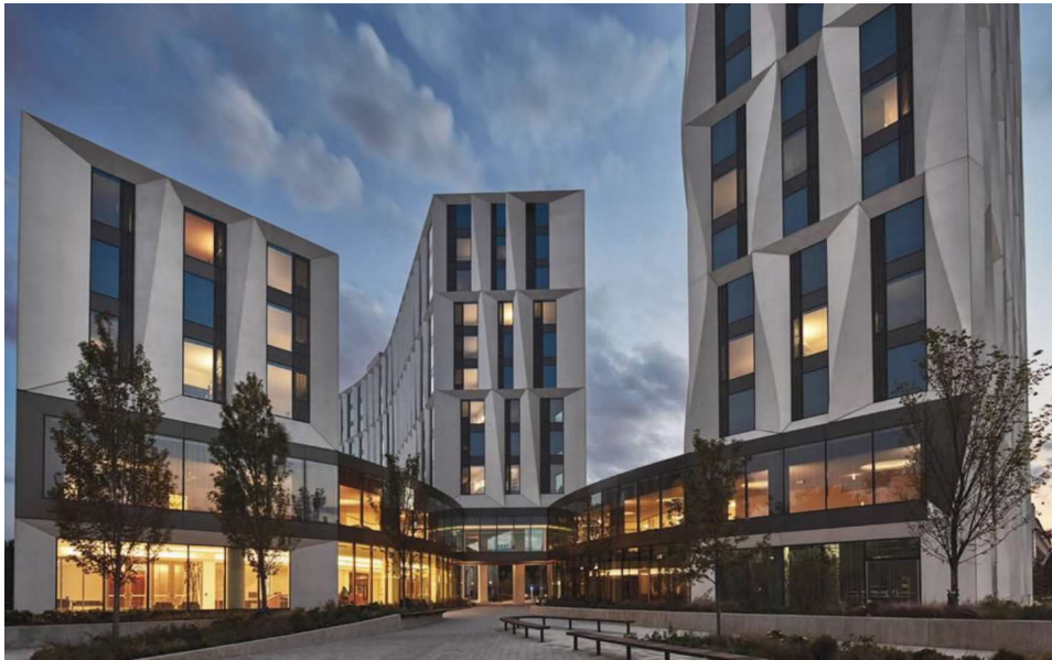
The University of Chicago Campus North Residential Commons feature student living quarters using REHAU in-slab hydronic radiant heating and cooling to improve energy efficiency and enhance comfort for the students.
