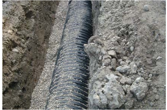
Fig. 07-3 RAUPIPEX pipe in a trench
